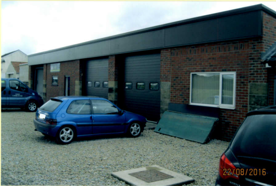
OLD COAL BUNKERS CONVERTED INTO CAR BODY REPAIR SHOP MR J GARDNER AND WOLF DIGS OFFICE AND WORKSHOP.
